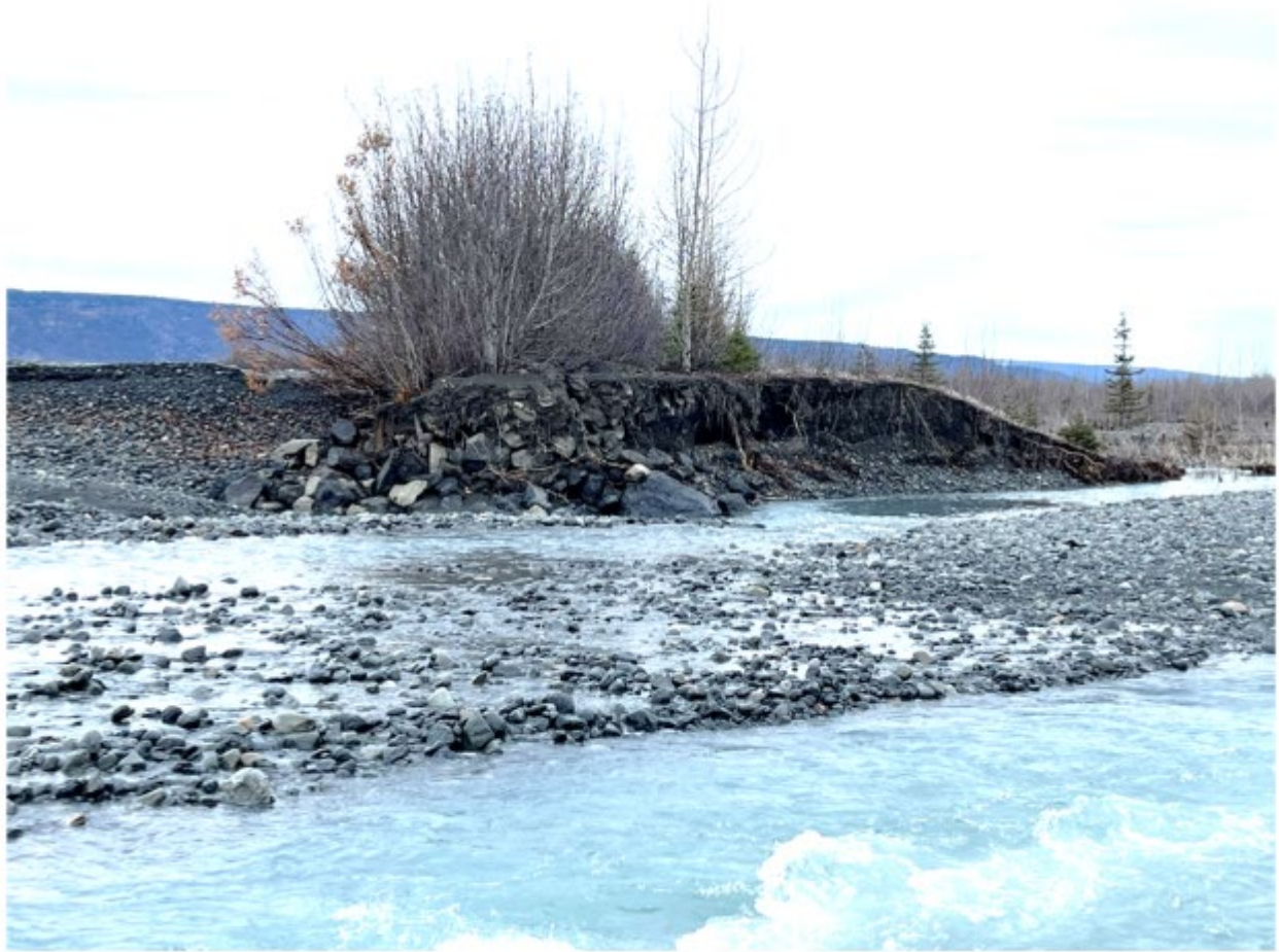
Photo 3-1 Cross-section of Levee at Breach Location November 2, 2023.
